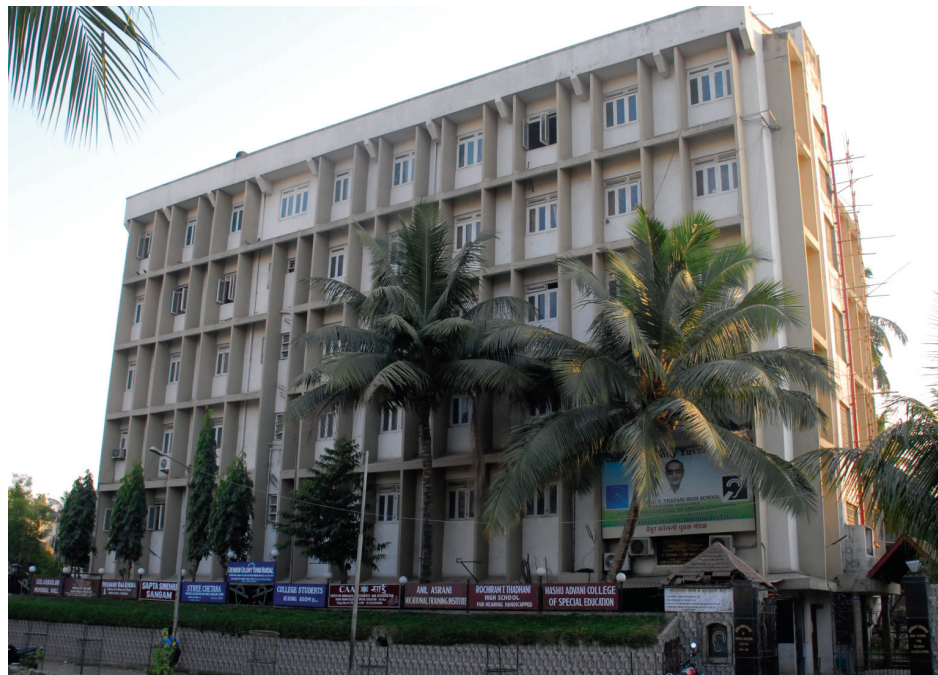
Chembur Colony, Yuvak Mandal Building, Collector Colony, Chembur, Mumbai
